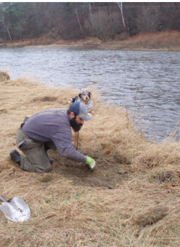
Planting live stakes along the Ammonoosuc River in Lisbon, NH – credit: NHDES Staff
