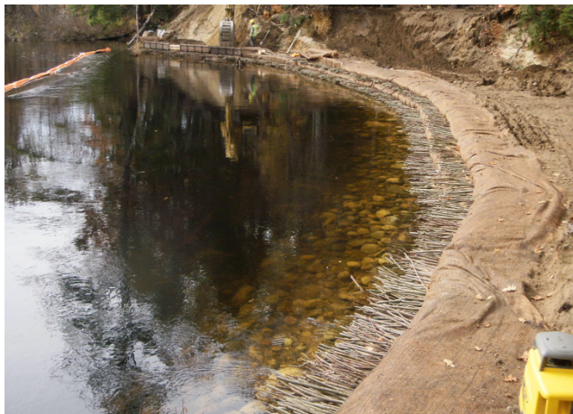
Streambank stabilization with brush layering during and post project – credit: Craig Rennie
