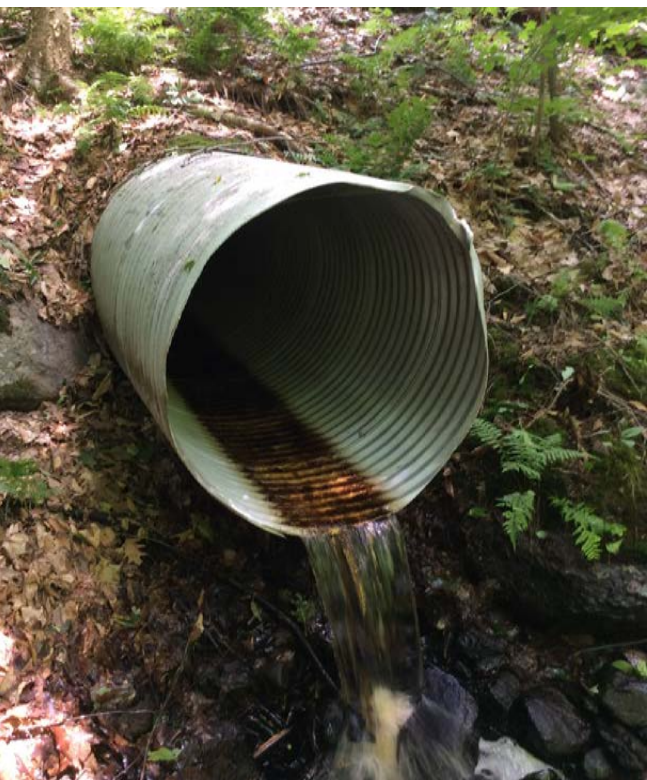
Perched culvert crossing under Sampson Rd., Rochester, NH – credit: NHGS
