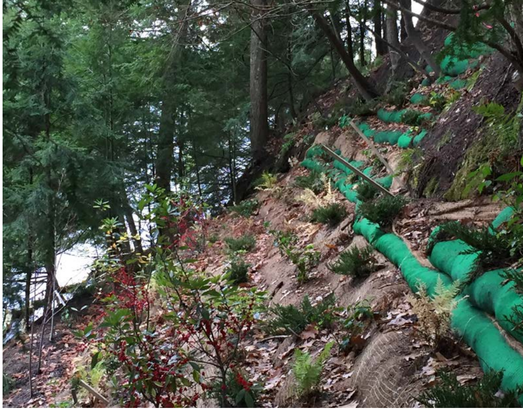
Slope stabilization using coir logs and live plantings – credit: Stefanie Giallongo
