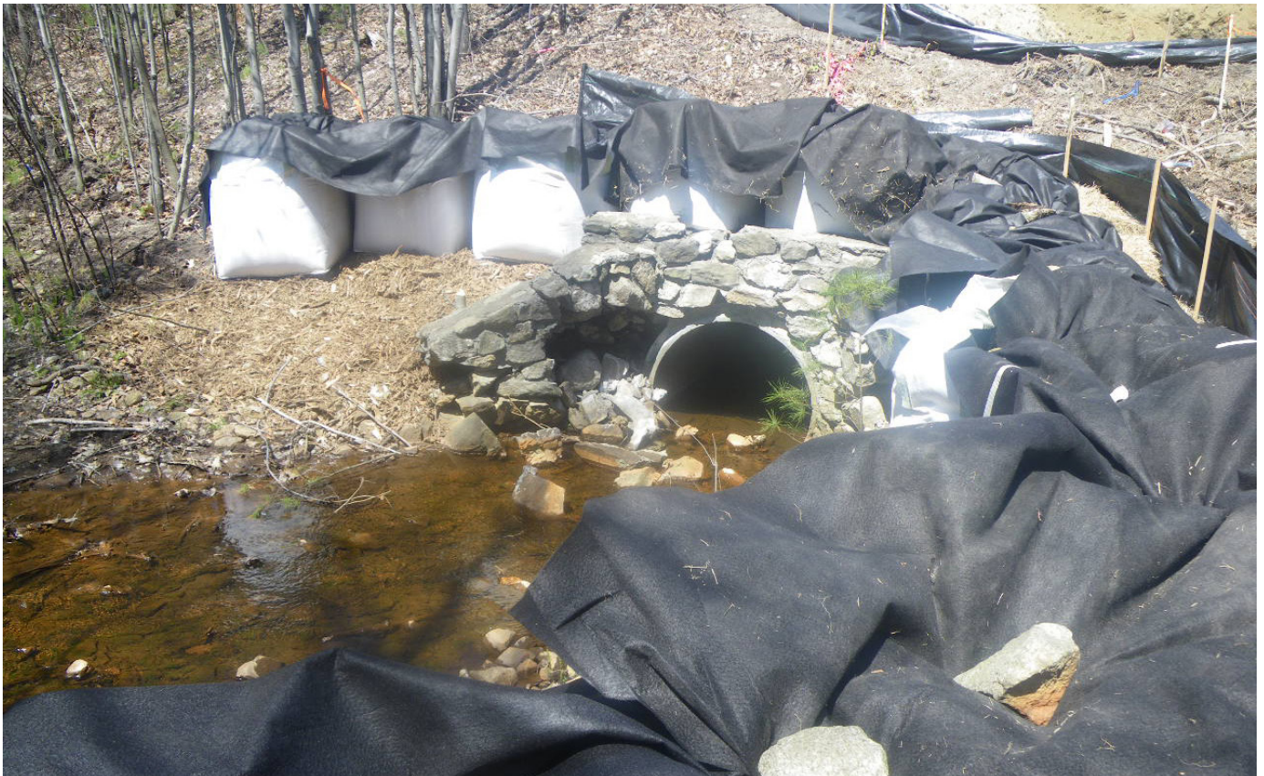
Erosion and sedimentation controls – credit: NHDES Staff
