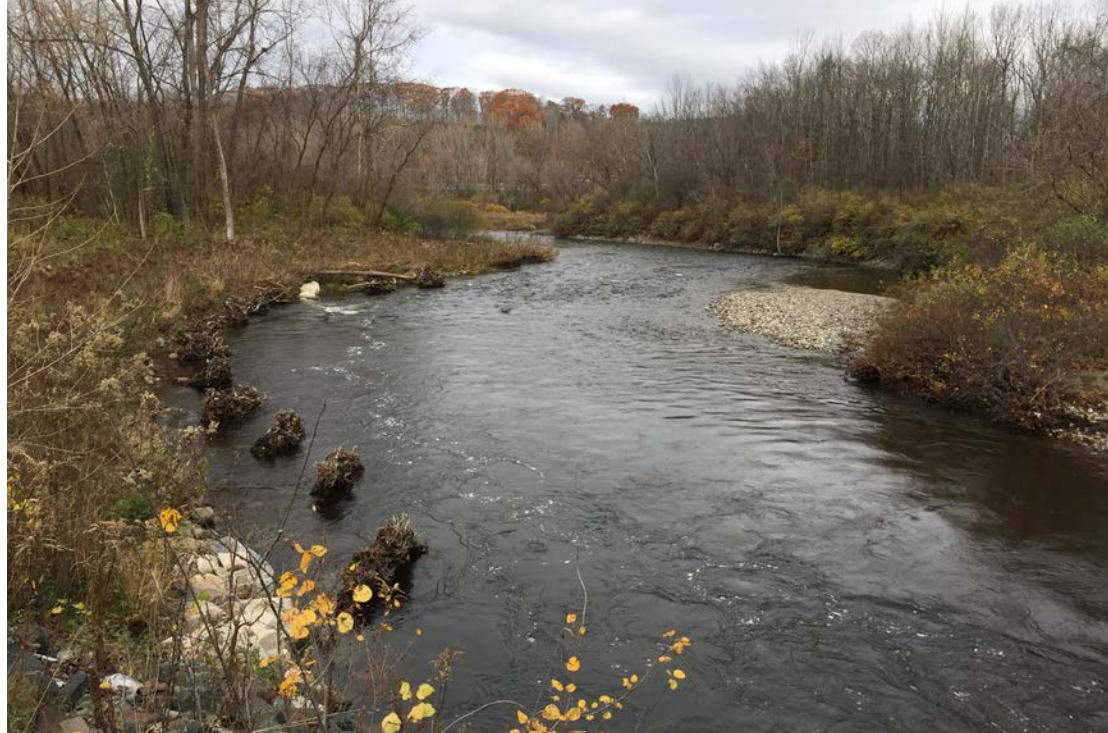
Root wad stabilization on Mascoma River, West Lebanon, NH – credit: Stefanie Giallongo
