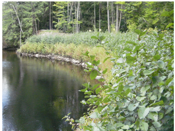
Streambank stabilization with brush layering during and post project – credit: Craig Rennie
