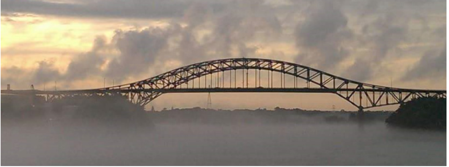
Piscataqua River Bridge, Portsmouth, NH – credit: Jay Aube
